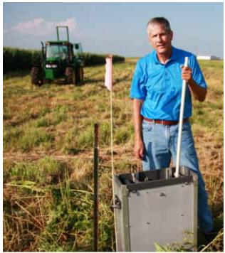
As a participant in the Mississippi River Basin Healthy Watersheds Initiative, Tim Smith installed a woodchip bioreactor in 2012 to reduce nitrate loads coming out of his tiled fields. Water from 30 to 40 acres can be diverted through the underground bed, which is composed of 125 cu. yd. of woodchips and permeable fabric, before flowing into a nearby stream. The flow of water can be controlled via stop gates. The Iowa Soybean Association both takes and examines the samples.
